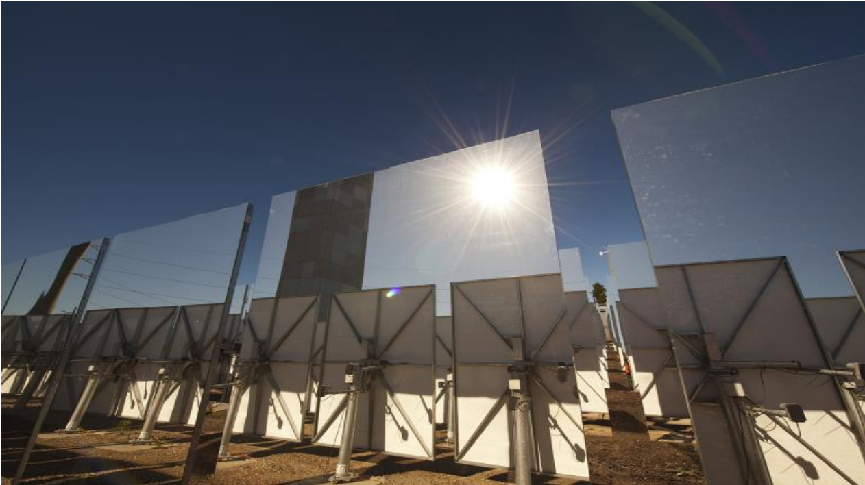
CSIRO's solar technology will be used for a heliostat field in Japan
